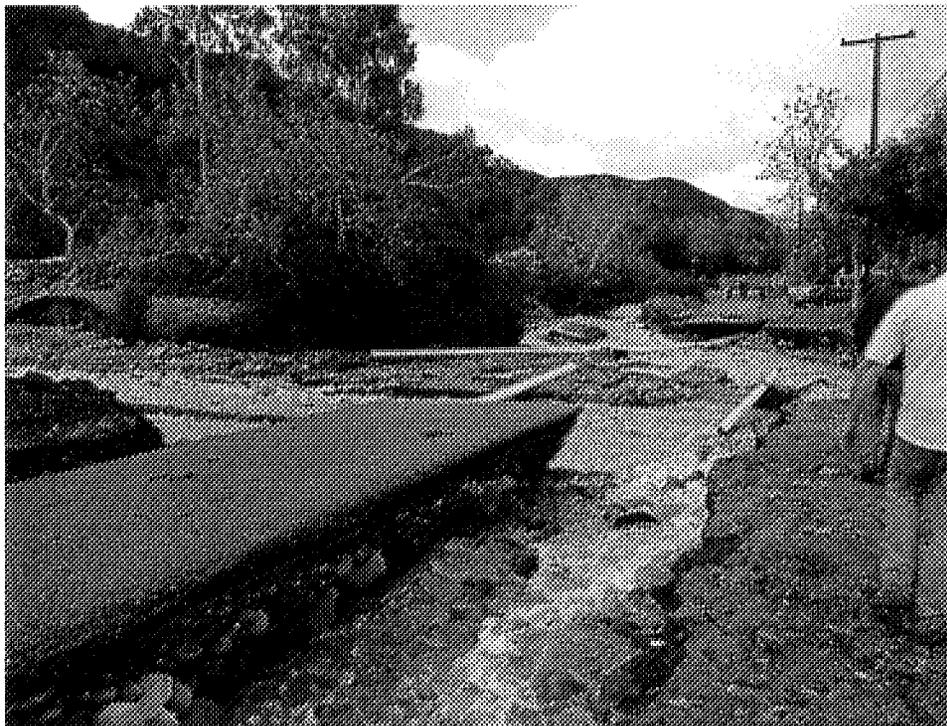
**Williams Canyon – Damage to Roadway and 8-inch PVC main near Creek Crossing (8-inch HDPE above-ground bypass constructed around this area)**
