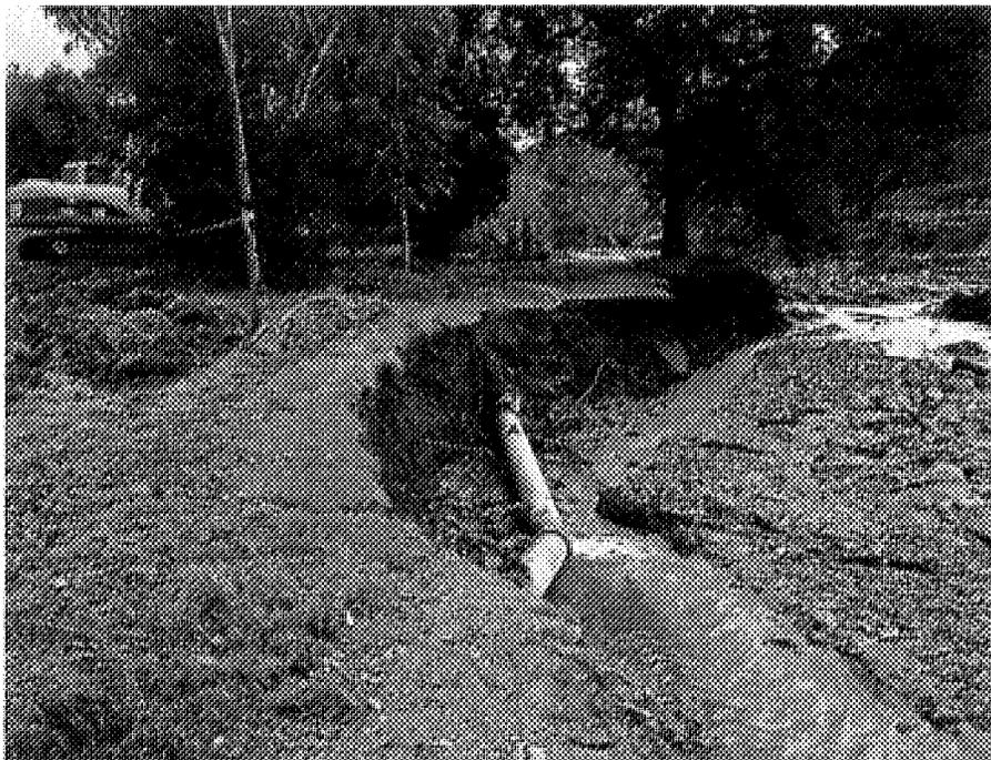
**Williams Canyon – Damage to Roadway and 12-inch ACP Main below Williams Pump Station (12-inch C900 bypass constructed around this area)**
