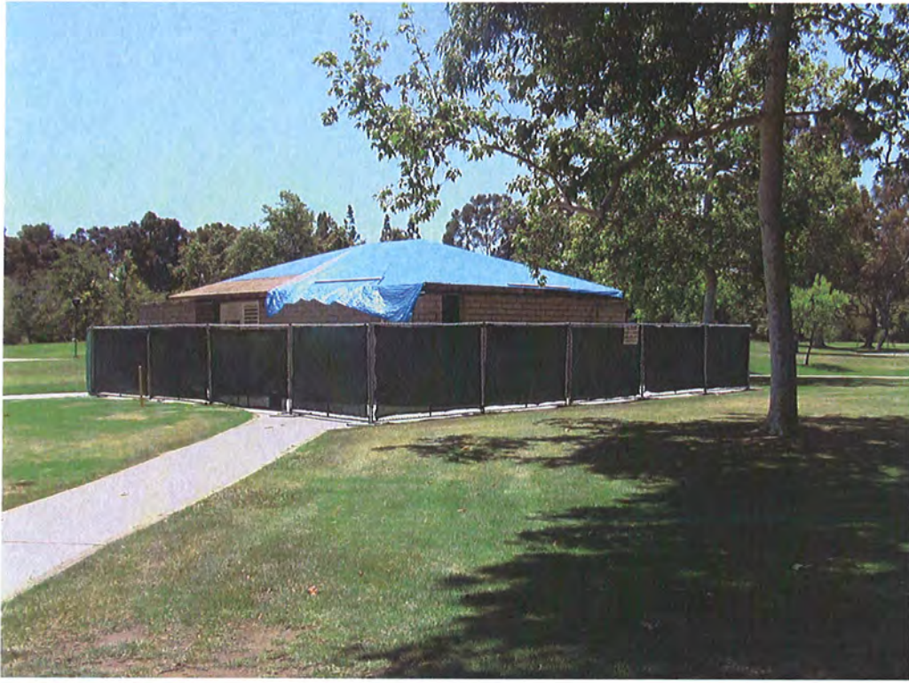
Photograph of Proposed Location No. 1 – Restroom Facility (currently under renovation)
