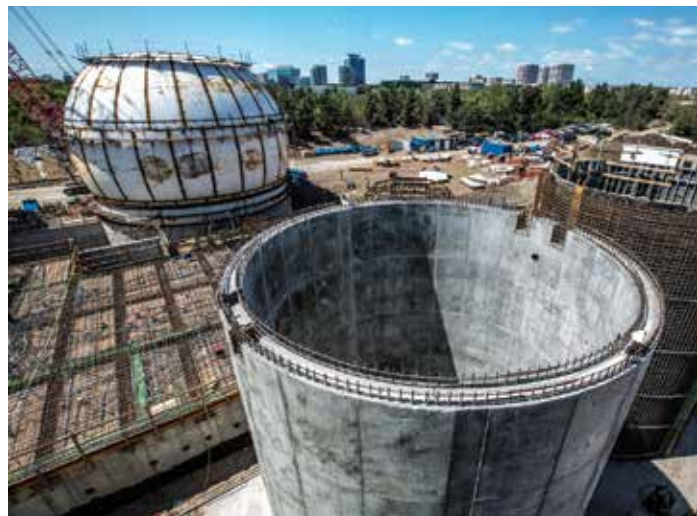
Biosolids and Energy Recovery Facilities Project
