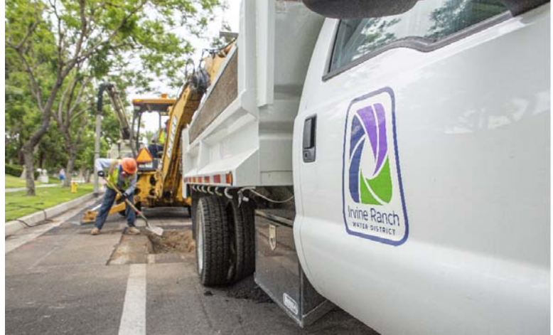
Field Crew on Site - Providing Essential Services
