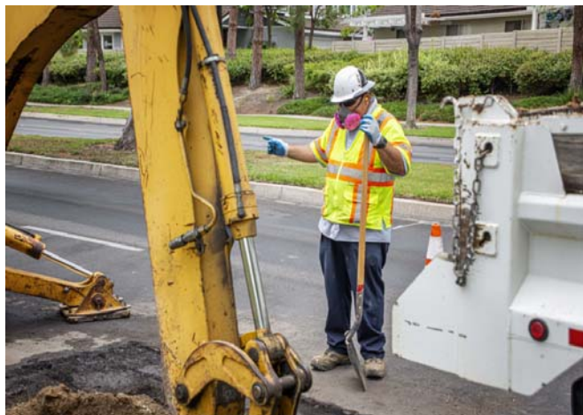
Field Crew on Site - Providing Essential Services
