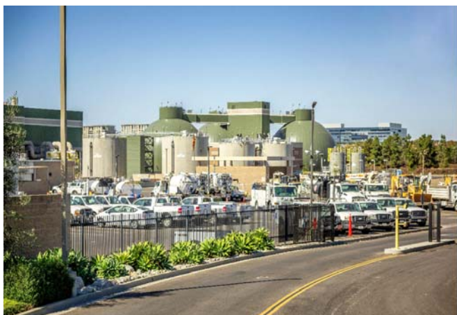
Biosolids and Energy Recovery Facilities
