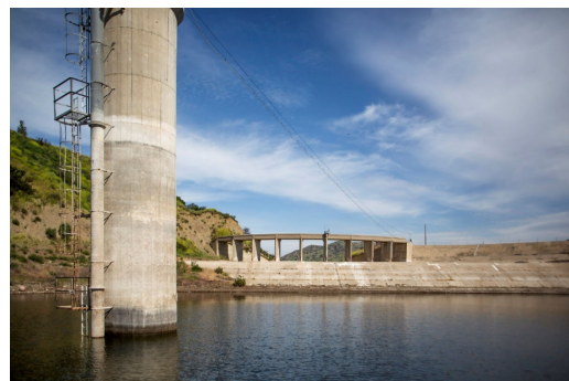
Santiago Creek Dam
