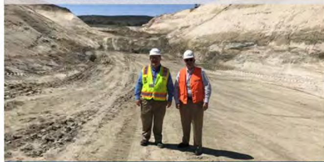
Mike Smith and Joe Ehasz at Trampas Dam Foundation
