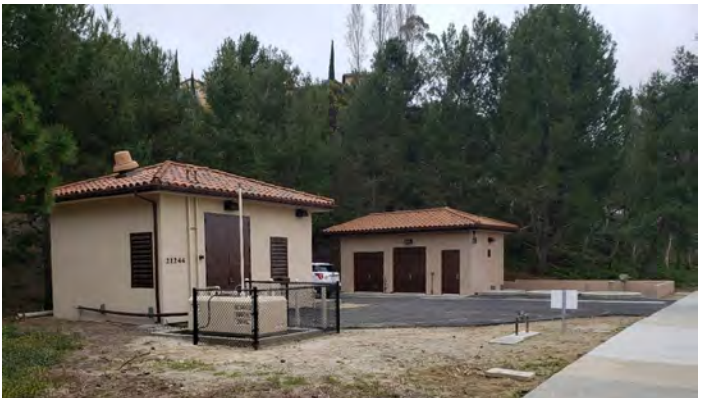
Figure 8: IRWD's Newport Coast Lift Station - Collaboration in Action. The GHD Team led by Greg Watanabe, our Principal-in-Charge, recently completed the design and construction of the abovenoted pump station. This is also a good example of collaboration with our subconsultants USI and TCE.
