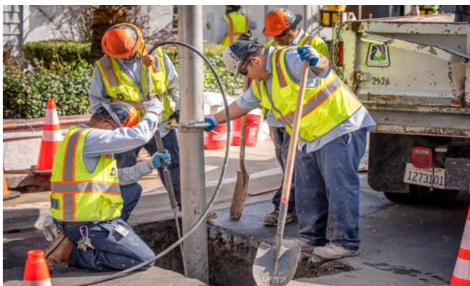
Field Crew on Site
