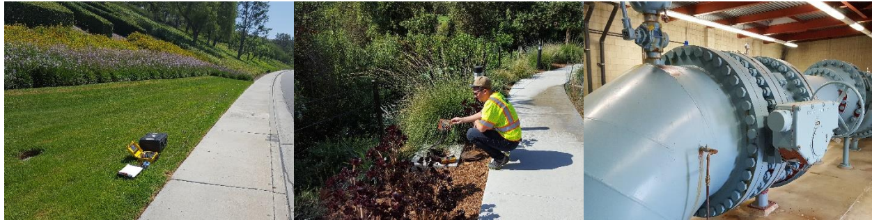
Electrical Continuity Testing
