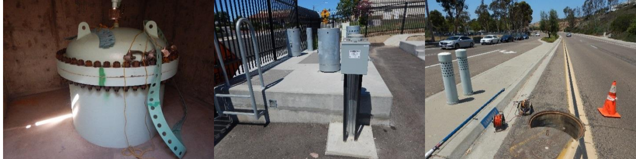
San Vicente Pipeline at Central Shaft
