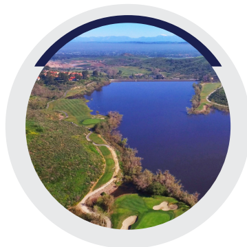
Sand Canyon Reservoir is one of four IRWD seasonal recycled water storage reservoirs.
