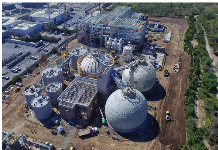
Biosolids and Energy Recovery Facilities Project
