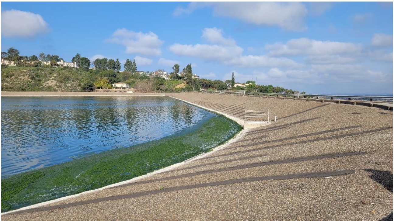
Photo 4: View of the upstream slope.
