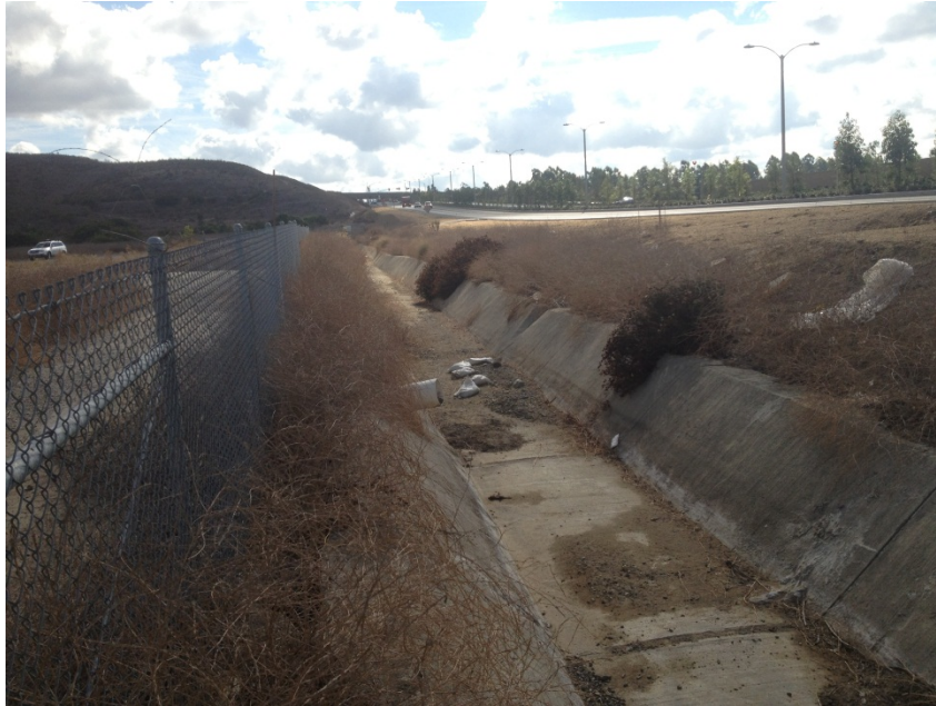
Exhibit E – Photograph is facing south and shows the concrete drainage structure adjacent to Portola Parkway
