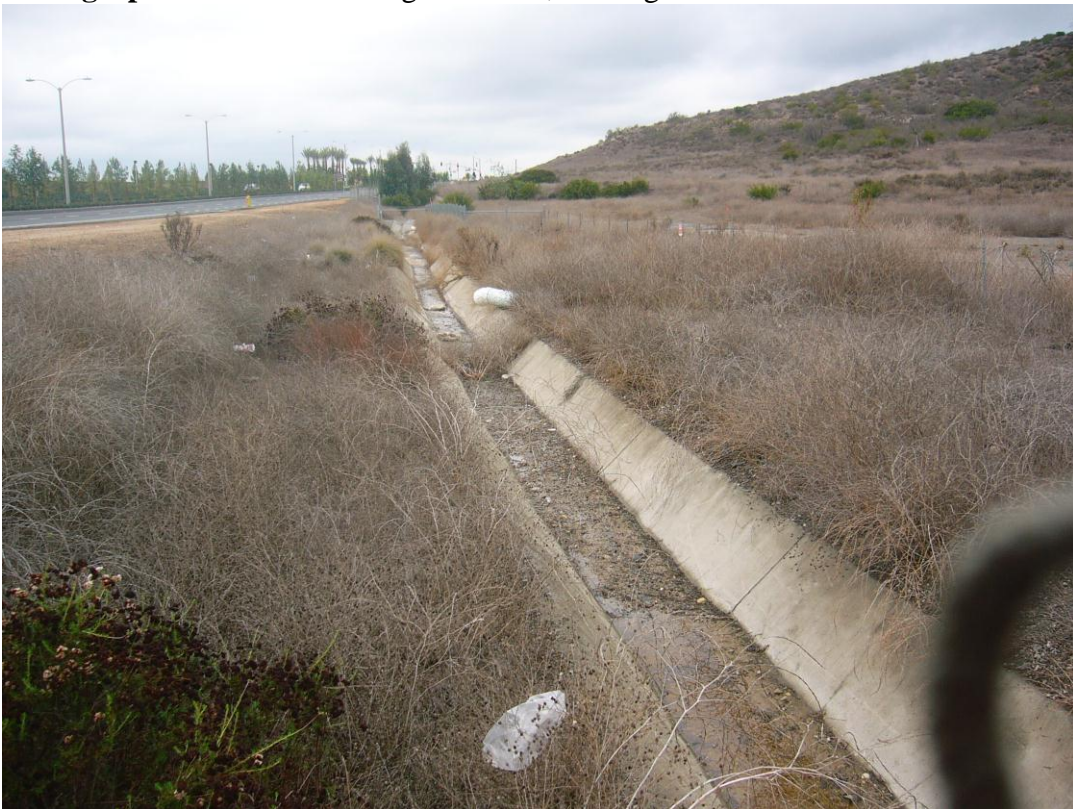
Photograph 2: Portola Drainage Channel, looking west.
