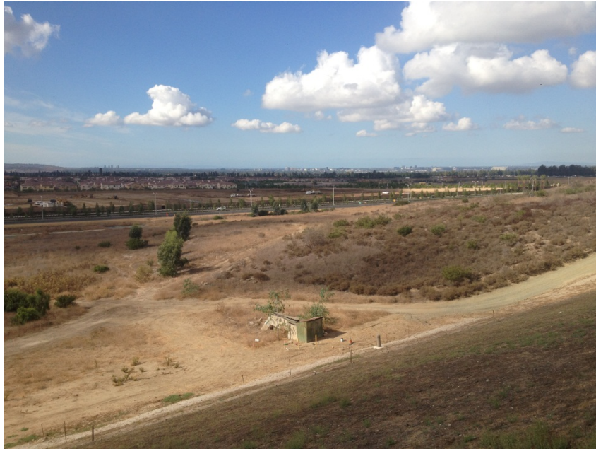
Exhibit A – Photograph is facing northwest and represents the project site (dam face is in the foreground)
