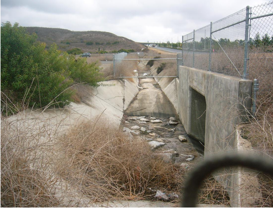
Photograph 3: Portola Drainage Channel, looking east at Portola Parkway culvert crossing.
