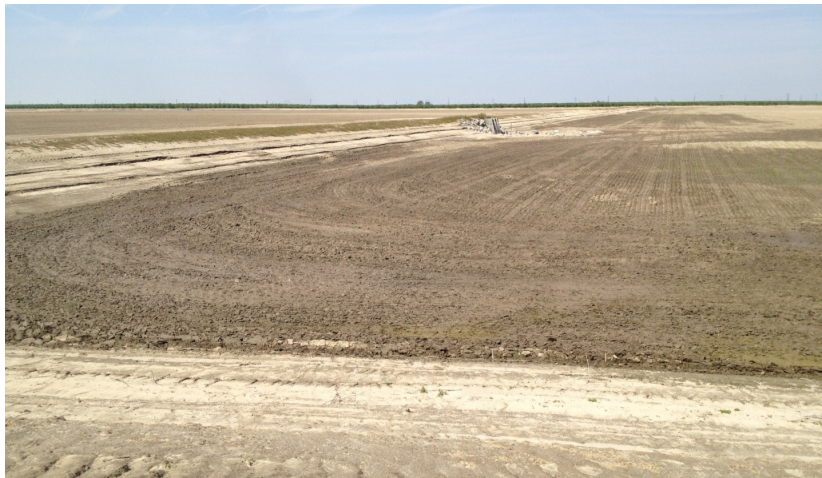
View of existing Stockdale West recharge basin
