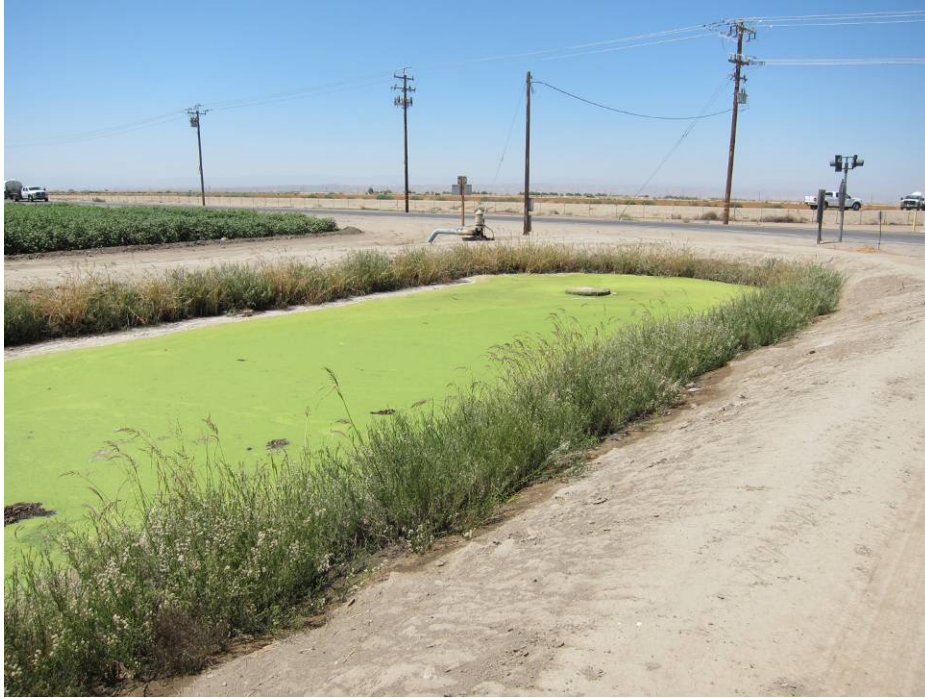
Photo 5 – Photo depicts the shallow vegetated water recharge basin in the northwest corner of the Stockdale East property
