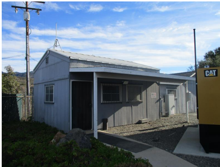
Figure 2. Office building: South (primary) and west elevation, view looking northeast (IMG_5886)
