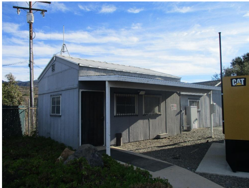
Figure 9. 7431 Santiago Canyon Road Office building: South (primary) and west elevation, view looking northeast (IMG_5886)
