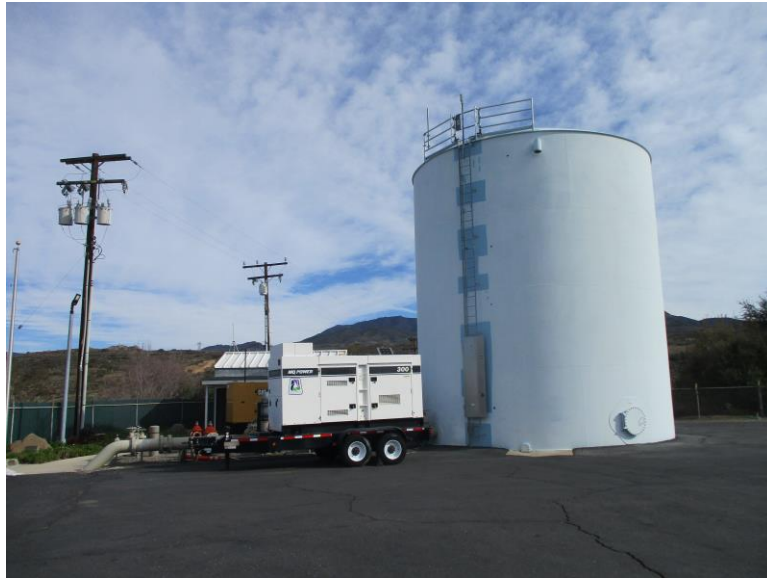
Figure 1. Reservoir, view looking north (IMG_5926)
