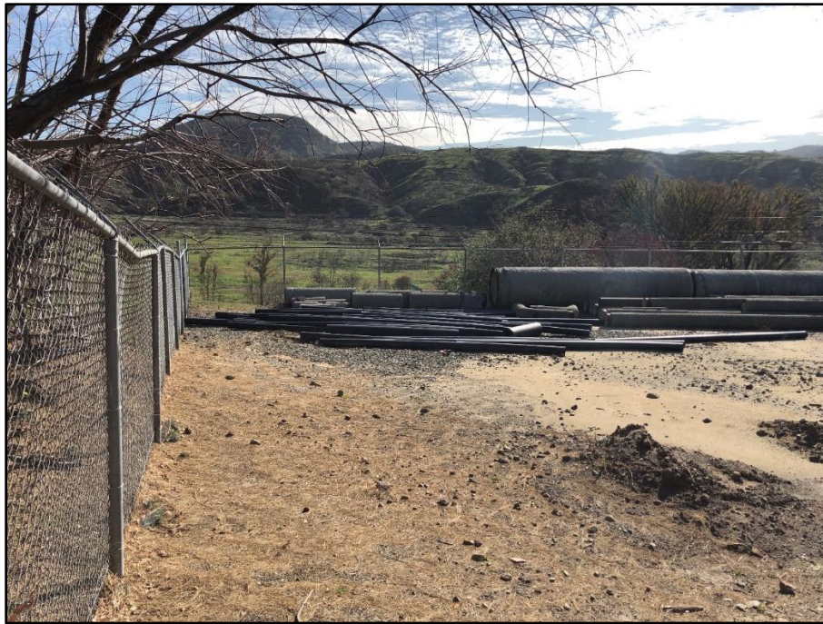
Image 1. View of Ground Surface Visibility within Dirt Lot Staging Area, Looking South
