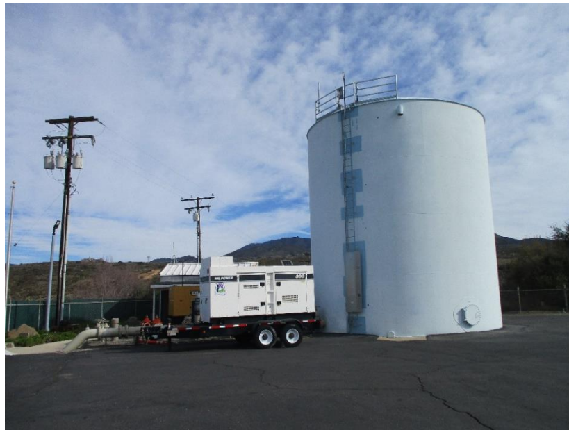
Figure 8. 7431 Santiago Canyon Road, Reservoir, view looking north (IMG_5995).
