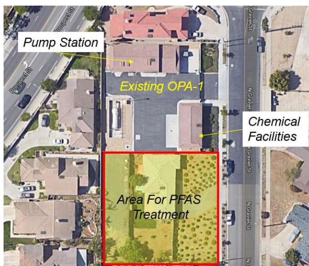
Figure 1-1: OPA-1 Existing Facilities and Area Designated for PFAS Treatment
