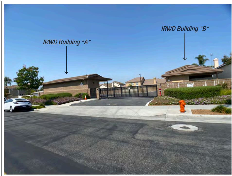
4-3a. View looking West from across North Gravier Street showing partial views of Building "A" on the left, the existing gate/driveway entrance, and Building "B" on the right.
