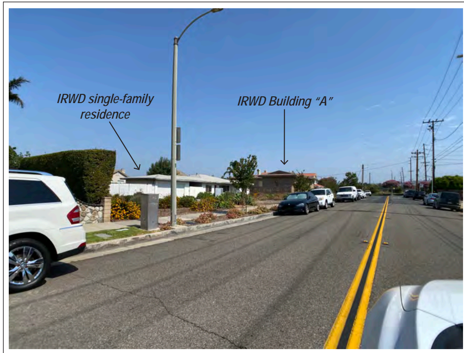
4-1a. View looking North on North Gravier Street towards the IRWD-owned residence and Building “A”.
