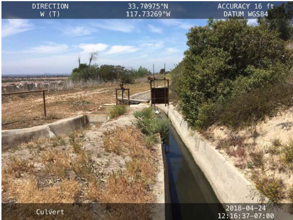
Photograph 10 -Photo west along the abandoned Highland Canal located in the southwest portion of the study area.
