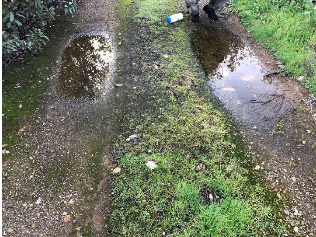
Photo 3: View of road rut puddle in access road on the west side of the reservoir (facing south).
