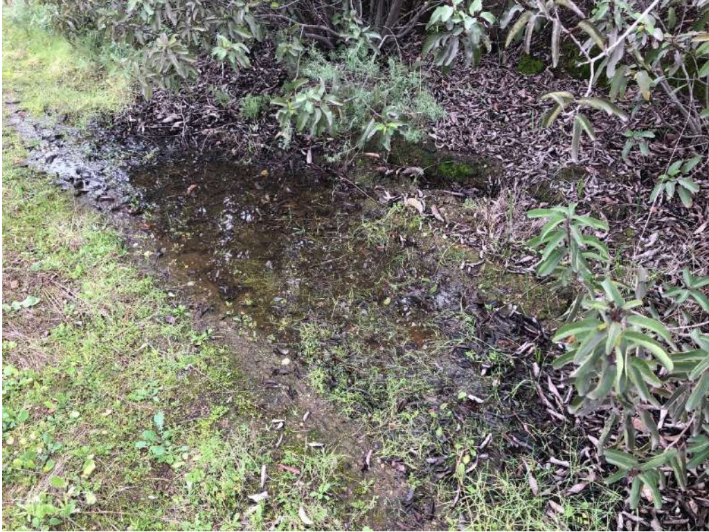
Photo 1: Puddle within the access road on east side of reservoir (facing northeast).
