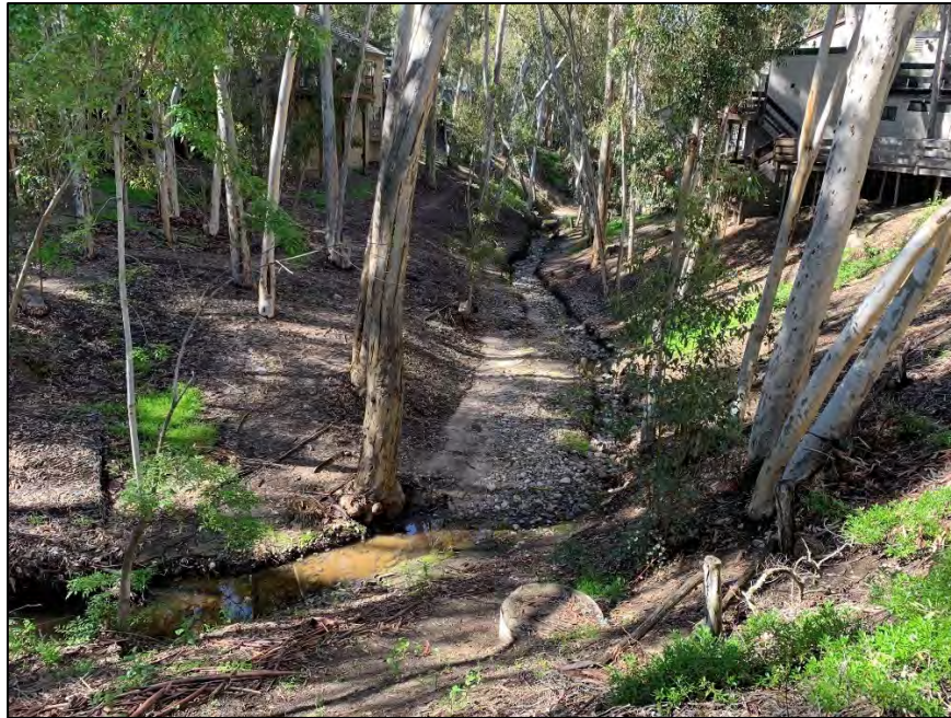
Photograph 3: Watershed improvement work area in the Glenwood Tributary. View to southwest.
