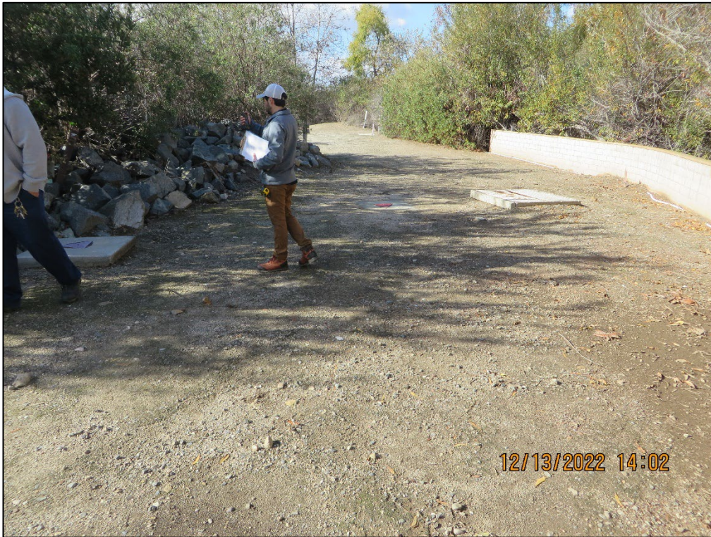
Photo 17) Location of downstream outlet control valves.
