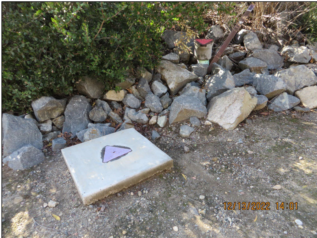
Photo 18) Location of downstream outlet control valves.
