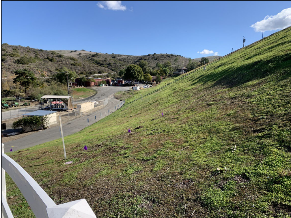
Photo 4) Downstream face looking towards right abutment.
