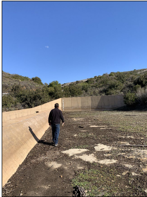
Photo 7) Close view of the spillway control ogee section and approach.
