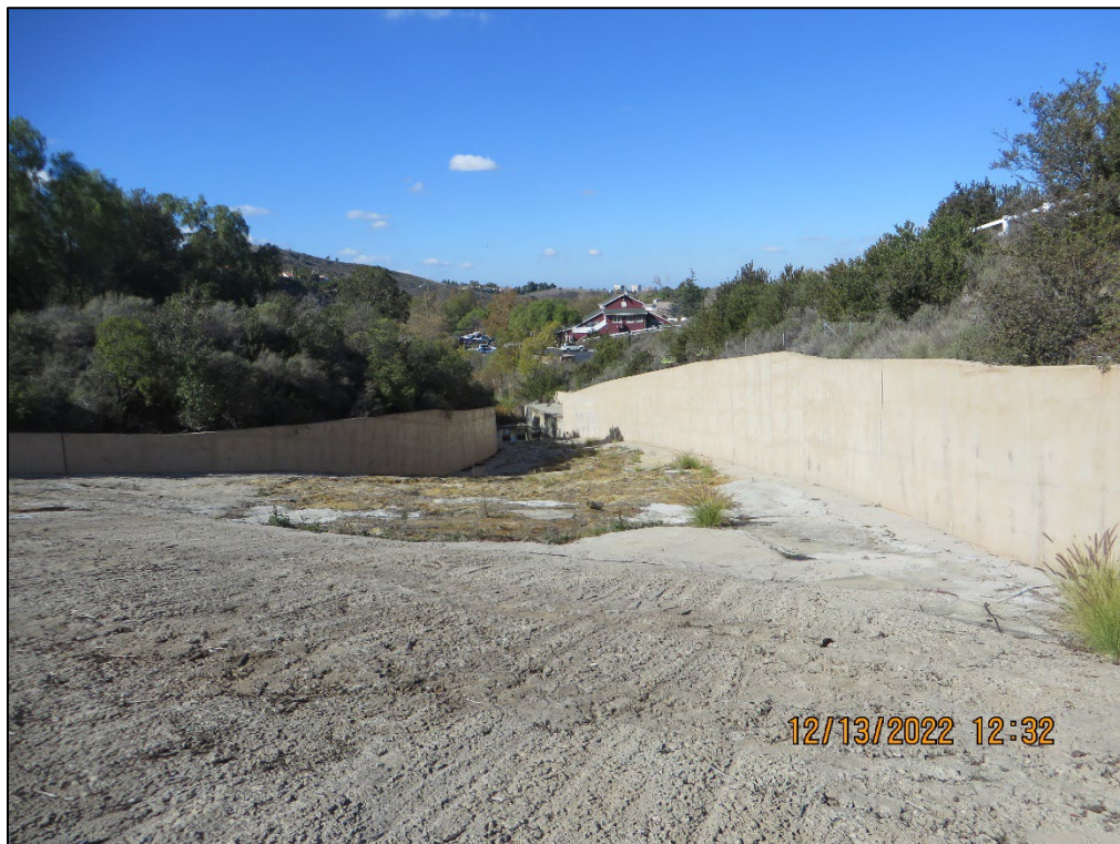
Photo 8) Spillway channel looking downstream.
