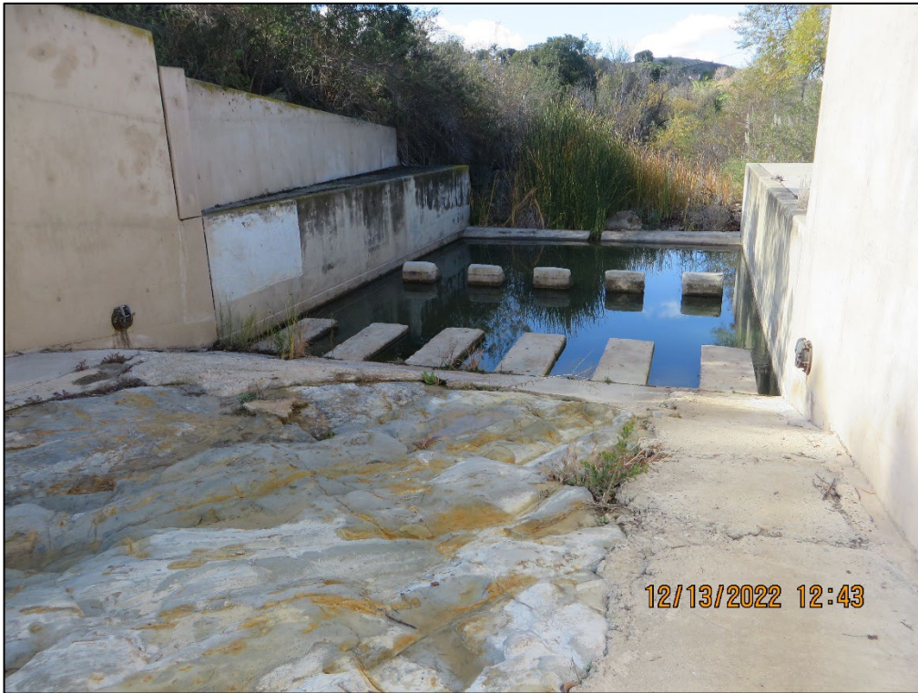
Photo 15) Close up view of spillway basin, note brush/tule growth downstream.
