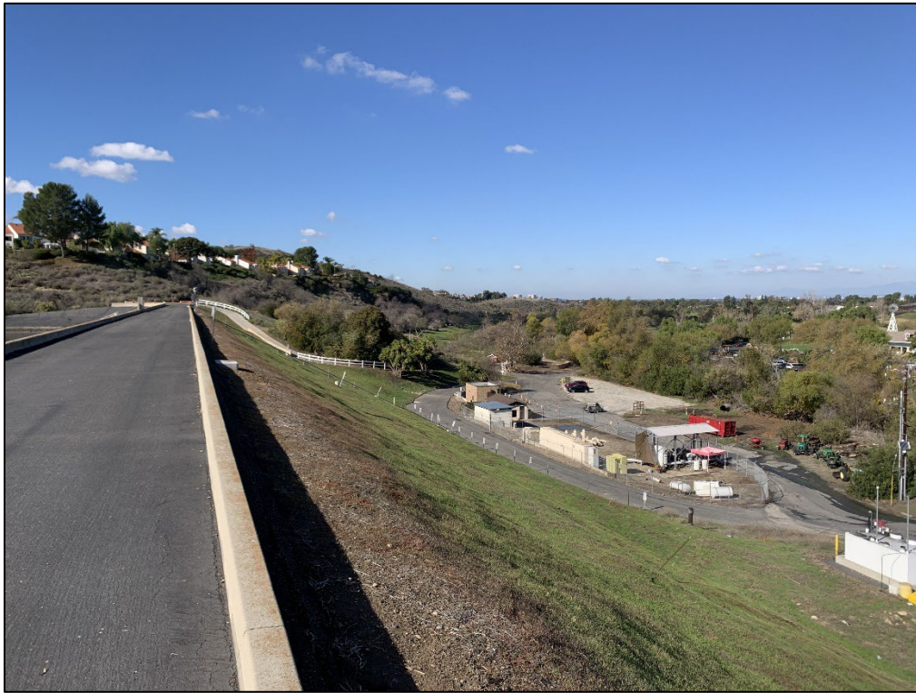
Photo 5) Downstream face looking towards the left abutment from dam crest.
