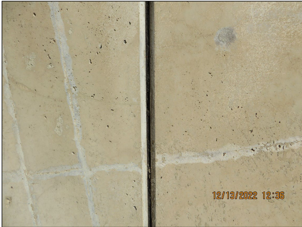
Photo 11) Close up view of expansion joint material between the spillway panels.
