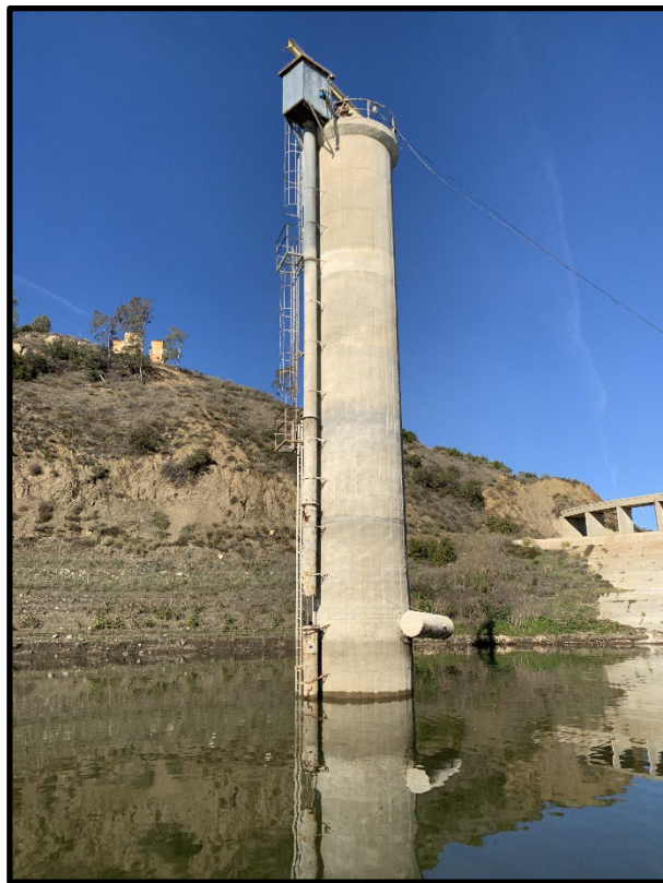
Photo 14) Concrete outlet tower.
