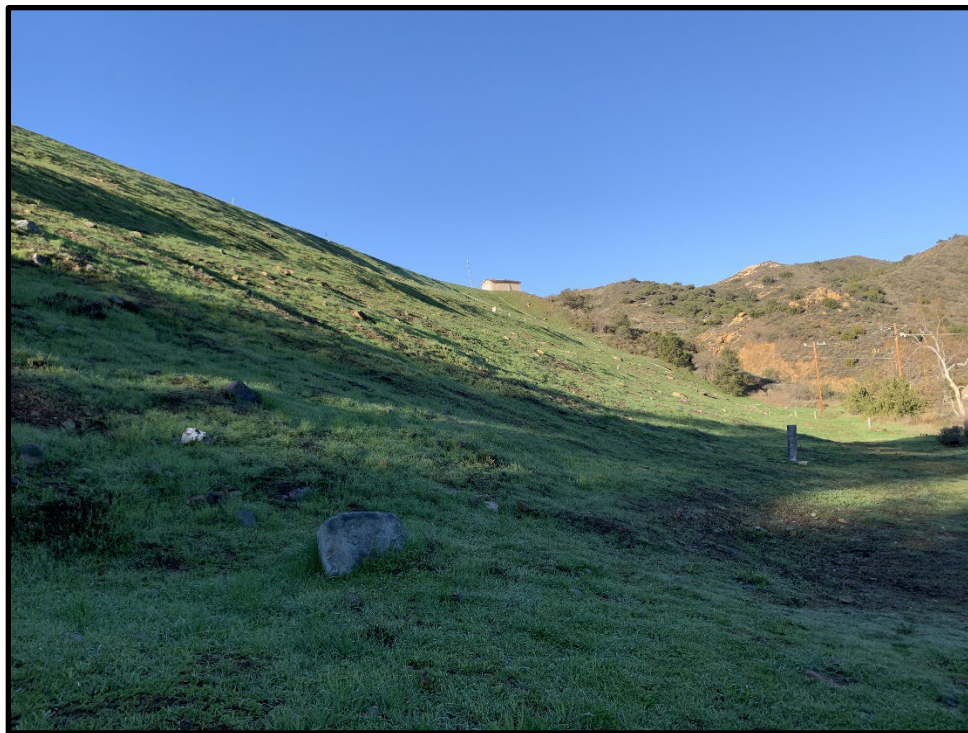
Photo 2) Downstream face looking towards left abutment area.
