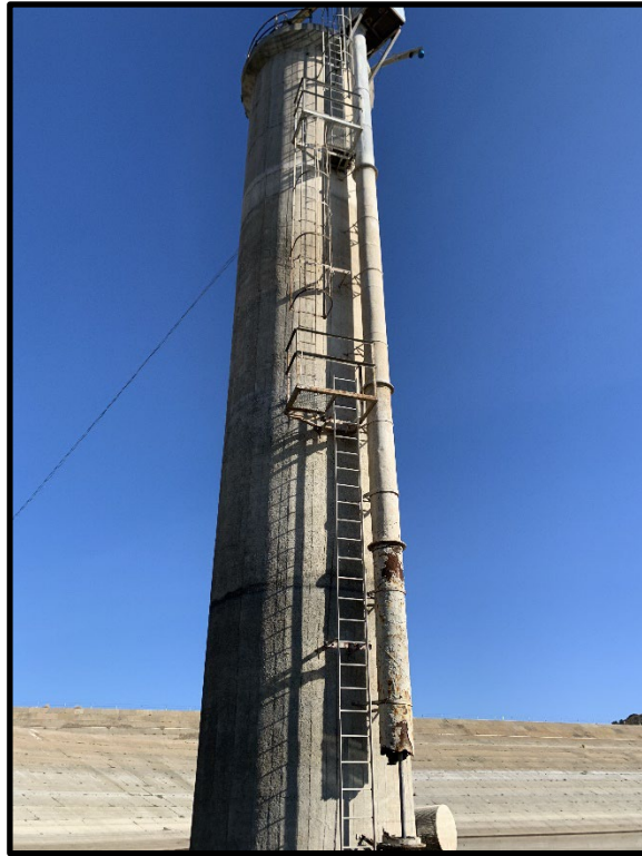
Photo 15) Concrete outlet tower.
