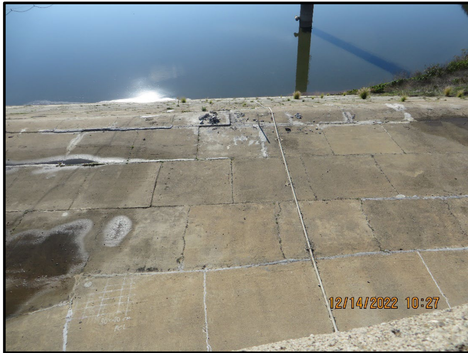
Photo 7) Recent concrete patch work on the spillway approach concrete panels.
