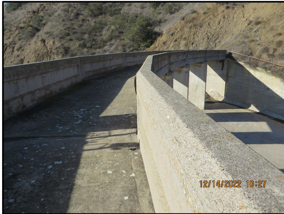
Photo 9) Spillway concrete bridge, piers, and chute looking toward left abutment.
