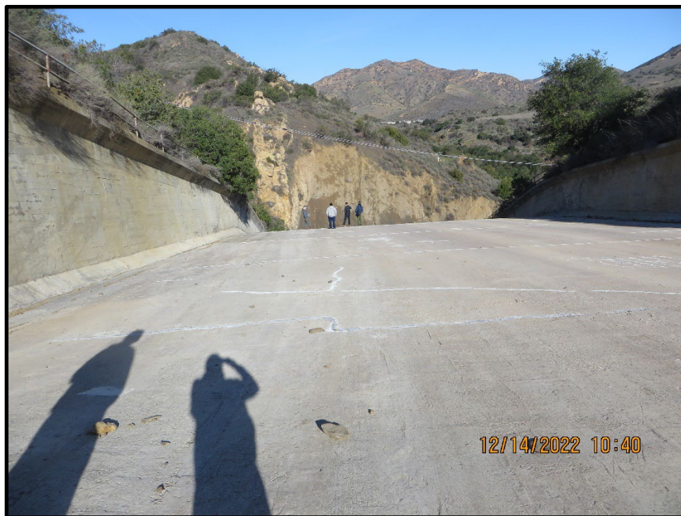
Photo 10) Spillway chute, looking downstream.
