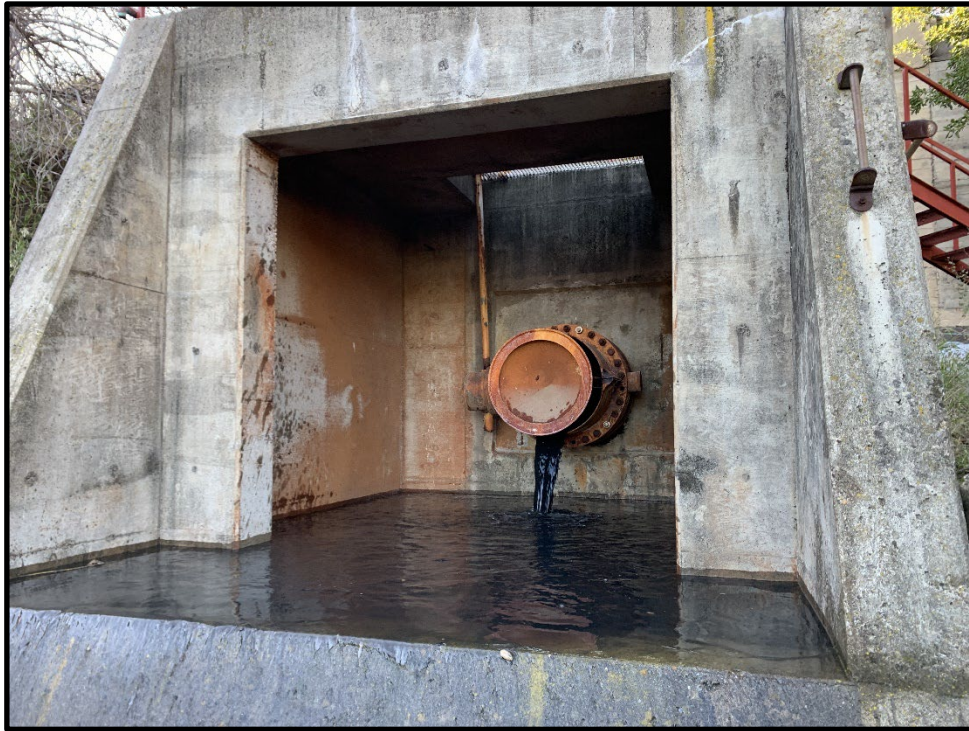
Photo 13) Emergency blowoff valve within dissipator structure. Note water flowing out.
