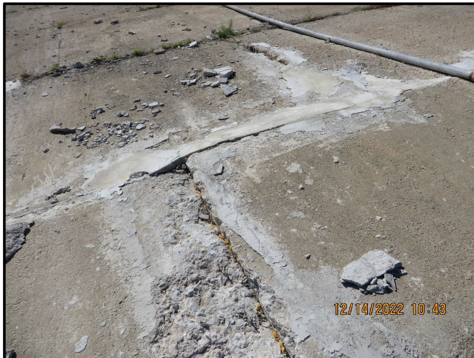
Photo 8) Recent concrete patch work on the spillway approach concrete panels.
