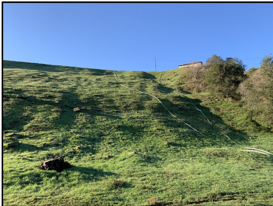
Photo 4) Downstream face looking towards left groin.
