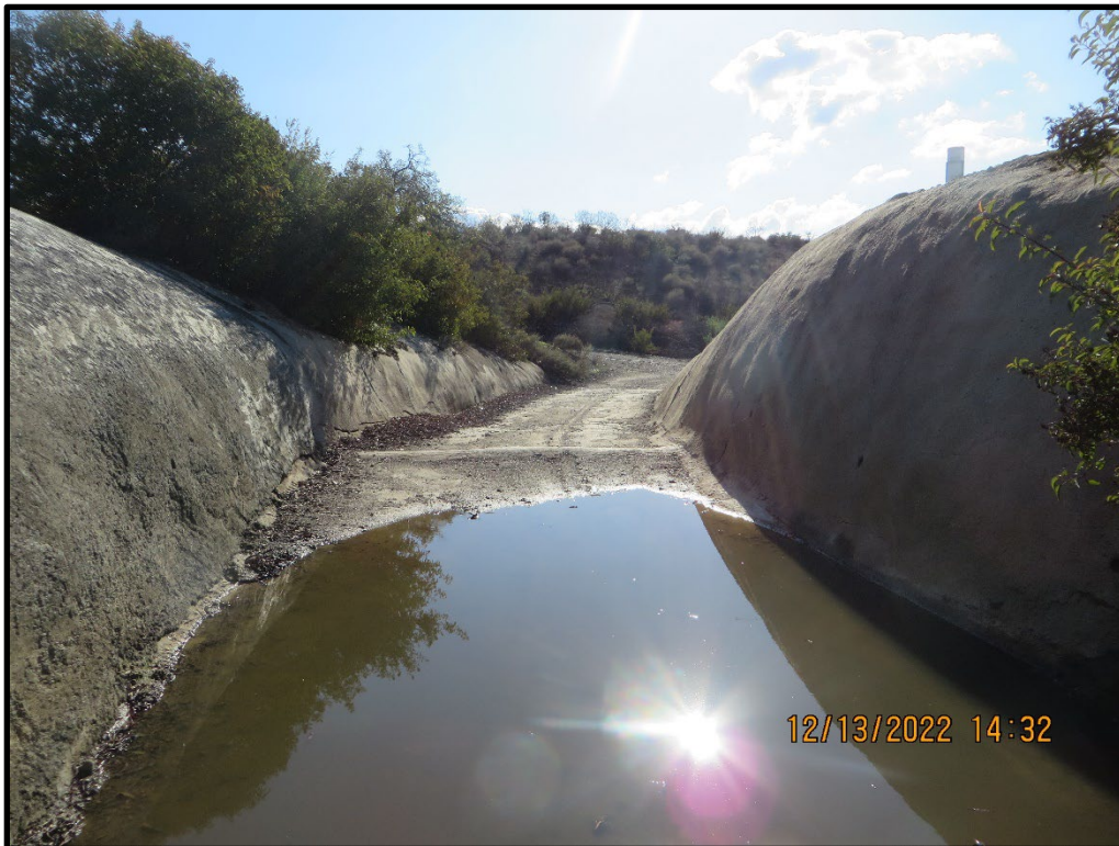
Photo 8) Spillway channel looking downstream.
