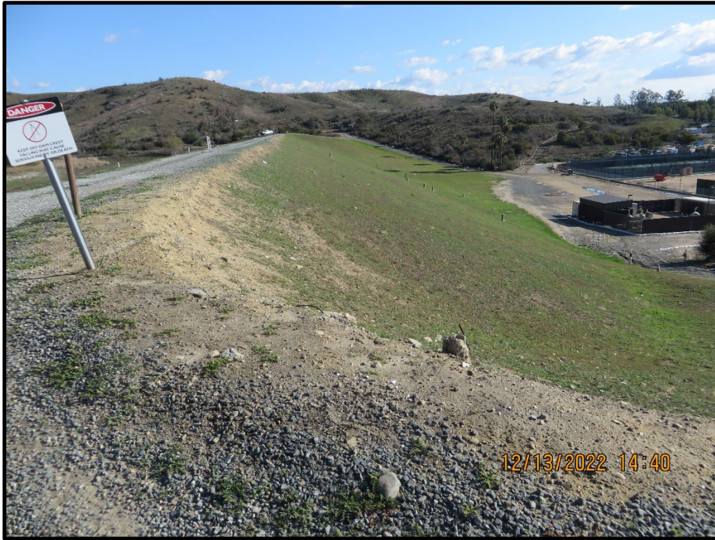
Photo 5) Downstream face looking towards left abutment.
