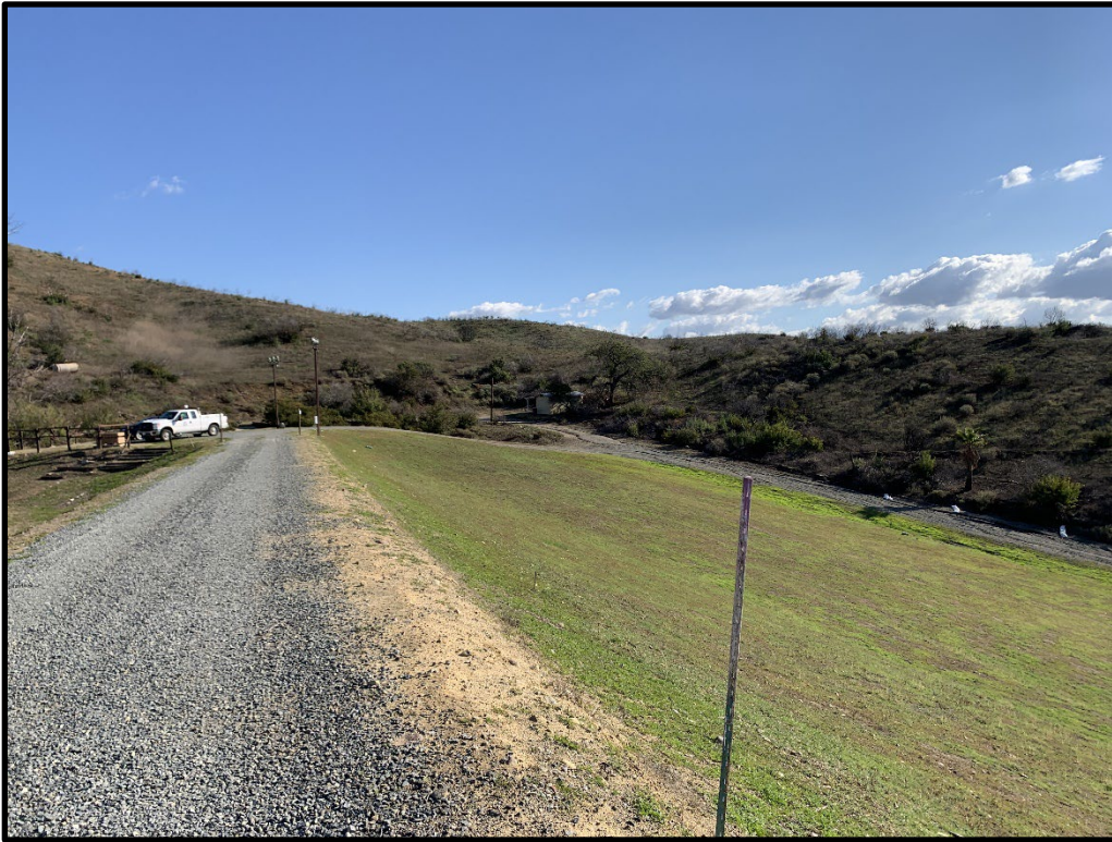
Photo 3) Crest and downstream looking towards left abutment.
