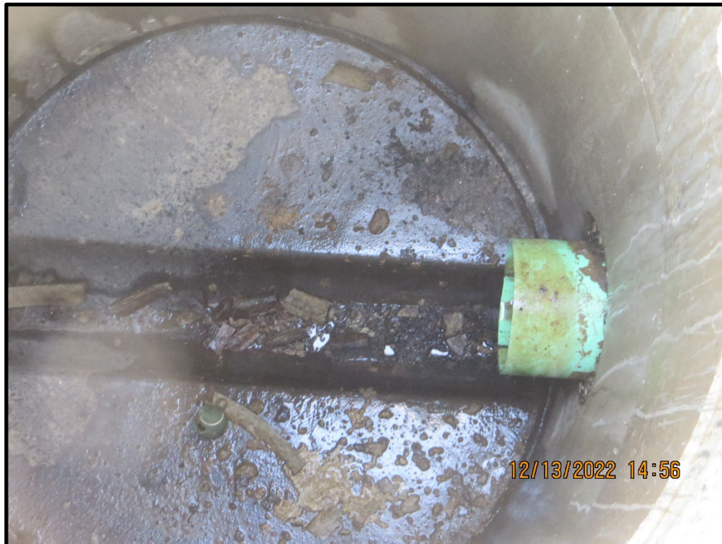
Photo 10) Drain outfall inside the seepage vault.
