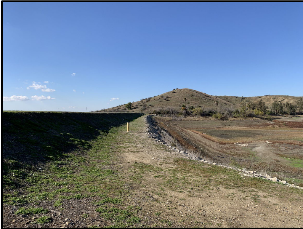
Photo 1) Upstream face looking towards right abutment showing bench and dry reservoir.
