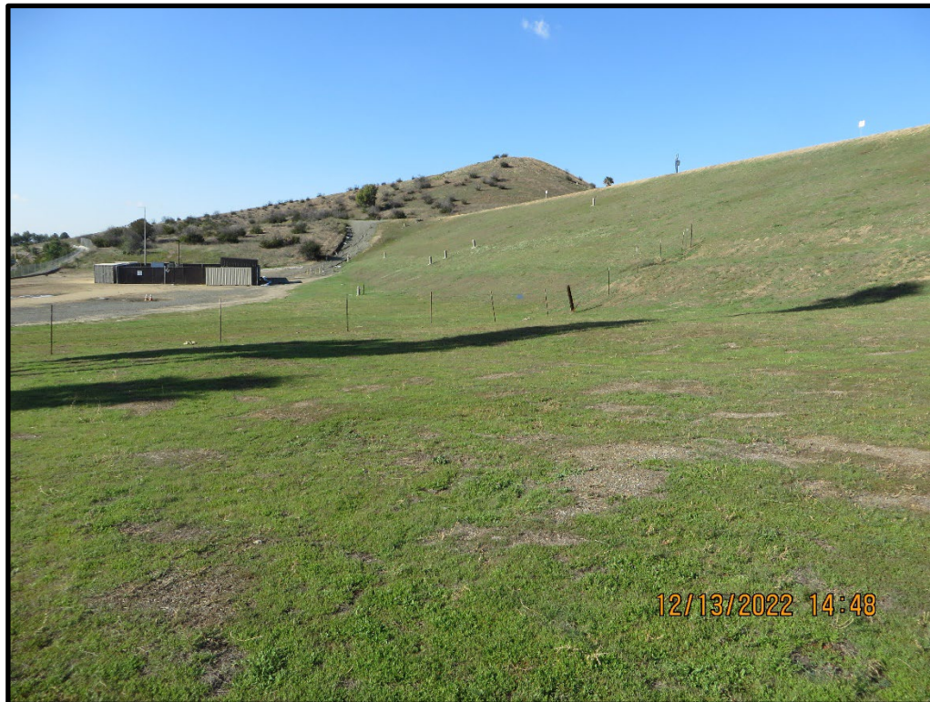
Photo 6) Downstream face looking towards right abutment.
