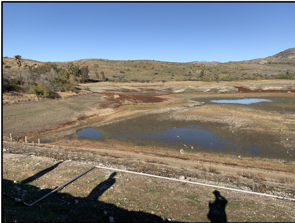
Photo 4) Dry Syphon reservoir.
