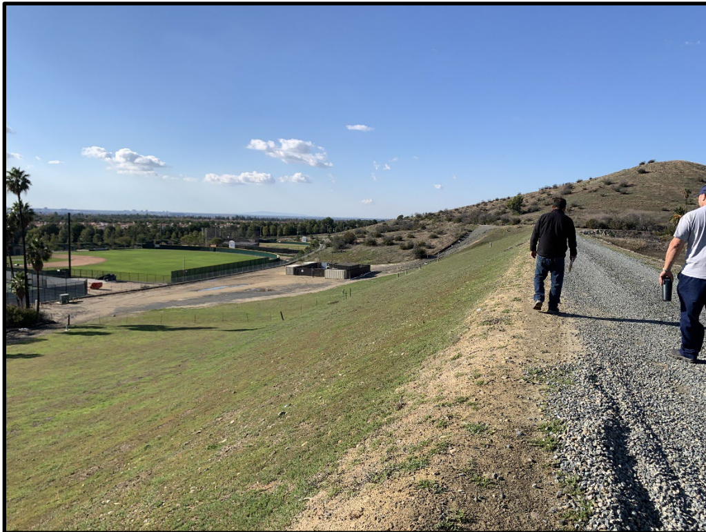
Photo 2) Crest and downstream face looking towards right abutment.
