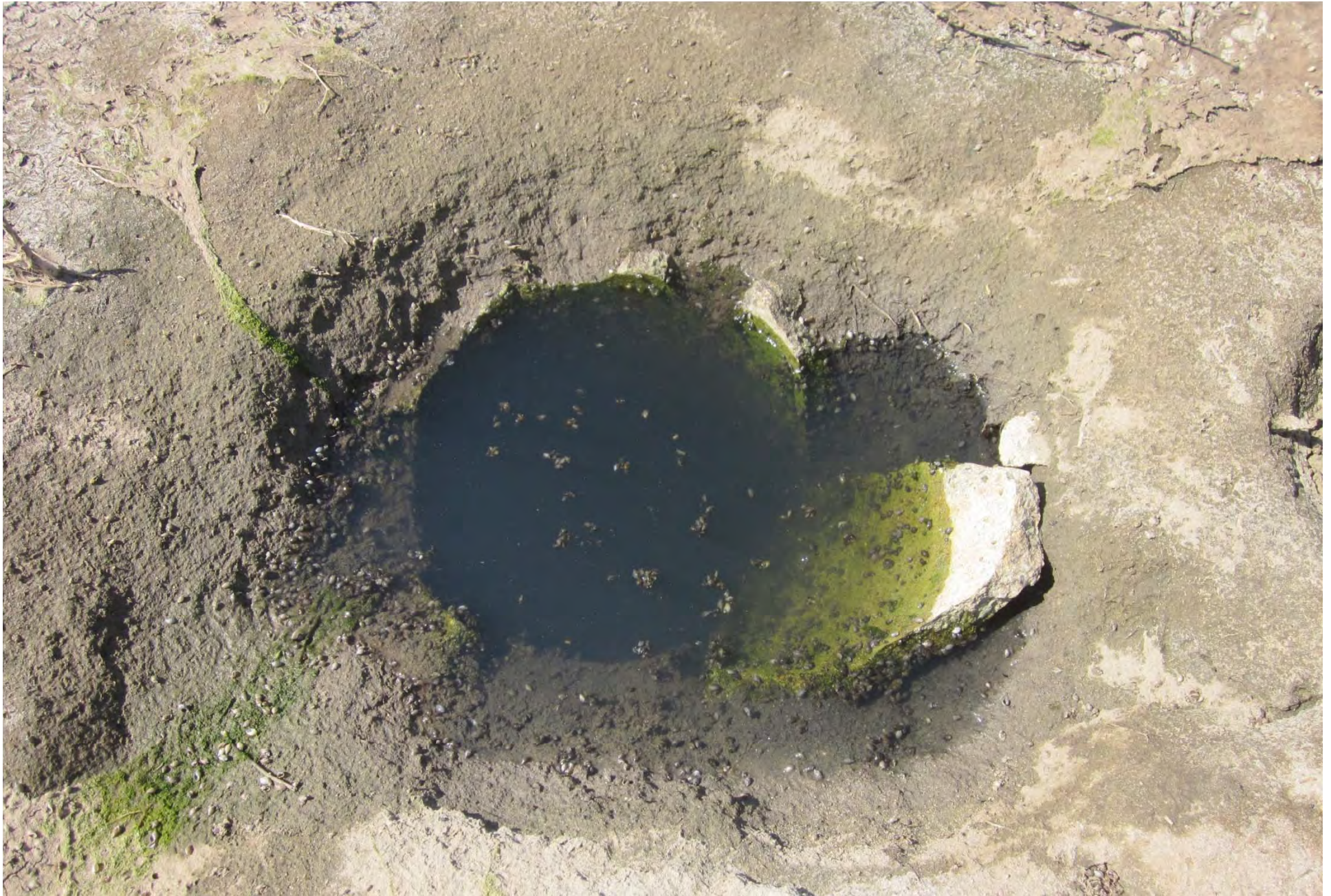
Photo 35 (5F): Old irrigated pipe filled with water in Basin No. 20; a second old pipe is barley visible to the right
