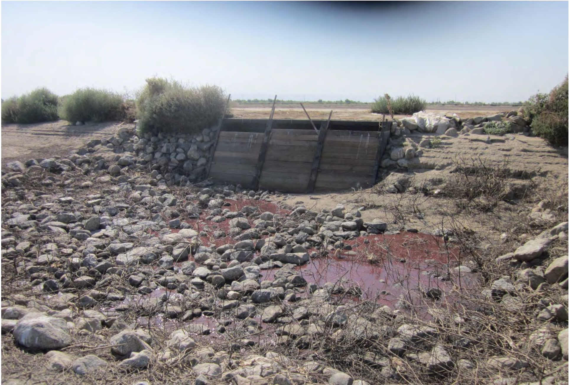
Photo 59 (22P): 3-Bay transfer structure between Basin No. 18 and No. 3; stagnant water in rip-rap with red algae and dead growth
