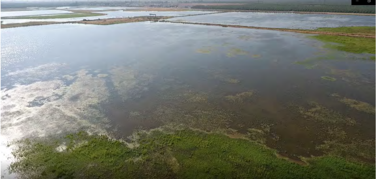
Figure 1. Example of a RRBWSD recharge basin with ponded water during the growing season that allows for the establishment of hydric soils and vegetation.
