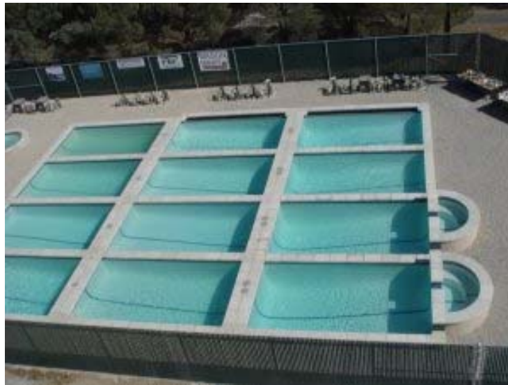
FIGURE 5. POOLS AND SPAS AT THE NATIONAL POOL INDUSTRY RESEARCH CENTER ON CAL POLY CAMPUS
