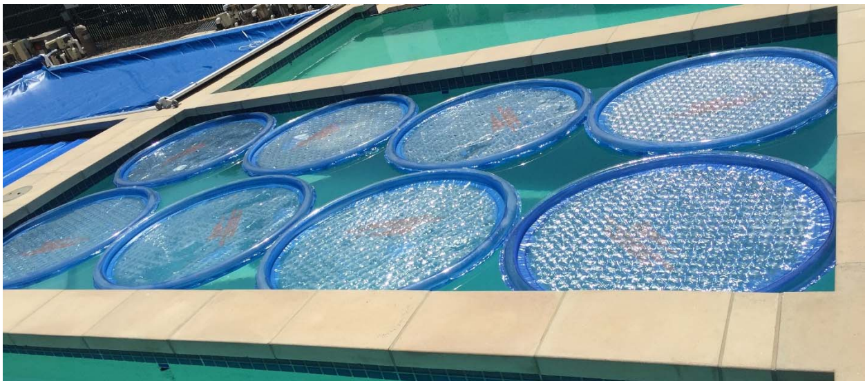
FIGURE 4. SOLAR DISKS INSTALLED ON A POOL AT THE NPIRC
